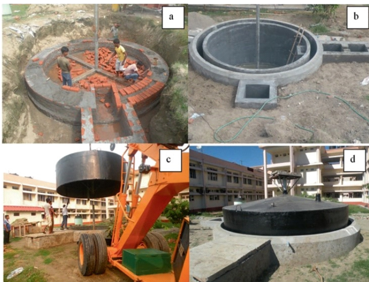
Figure: (a–d) Construction phases of the biogas plant
