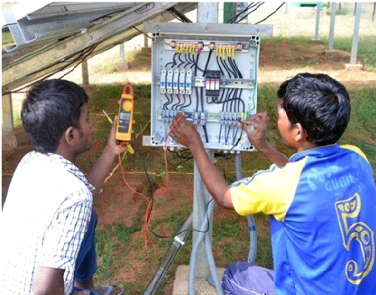
Fig: 10 Mini-grid operator and engineer testing the mini-grid power supply
