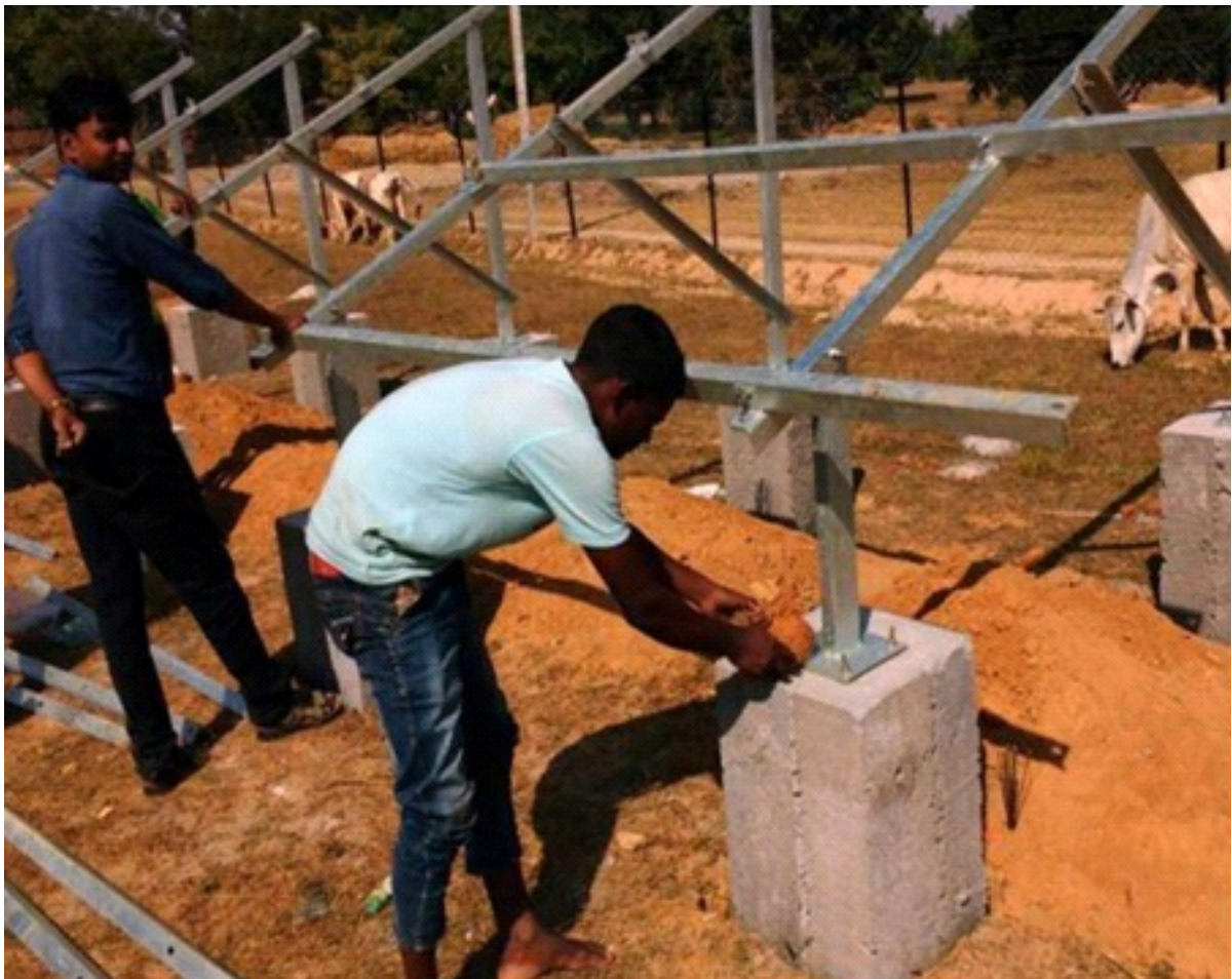
Fig: 6 Local workers installing the framing for photovoltaic solar panels (Source: Mlinda, 2019)
